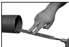
Figure 2: Deburr inside diameter using a half-round file
